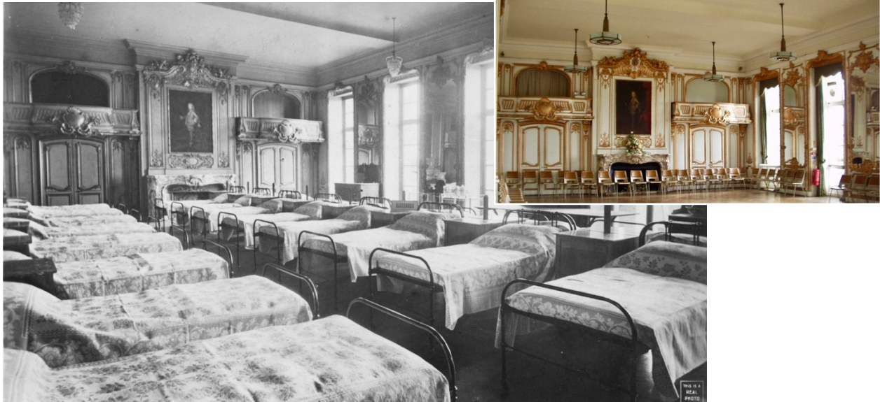
Above and inset: A postcard from 1914 of the Alexandra Ward, later the Paget Ward, formerly the ballroom and a colour image of the ballroom from recent times. [ americanwomenswarhospital.com/gallery/TOL008 ]
