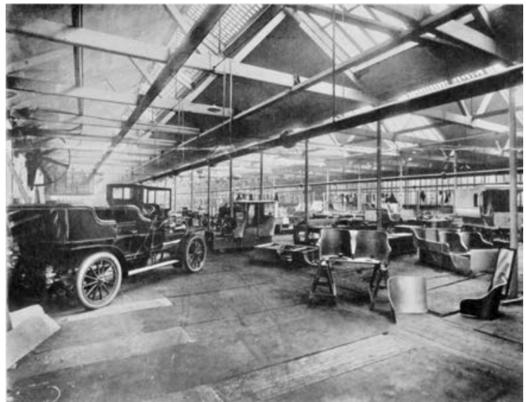
Right and above: A corner of the Argyll Motor Cars workshop in Glasgow illustrating the Roi-des-Belges stamped sheet metal panels and a completed car from their 1905 catalogue.
